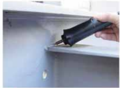
● Measuring the strength of welding sections (Checking tension strength)
