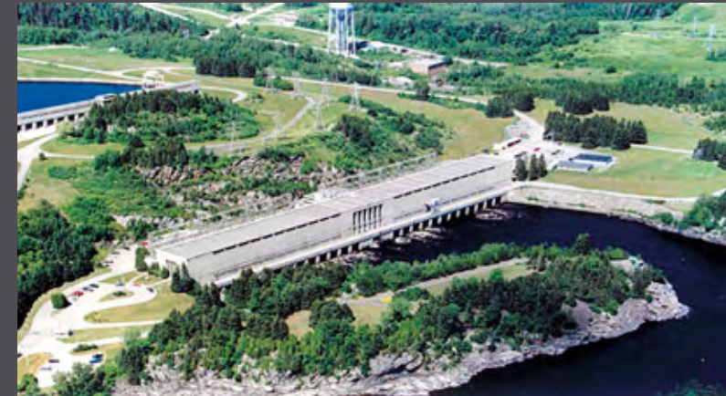
Shipshaw HPP (courtesy of Alcan Canada)
