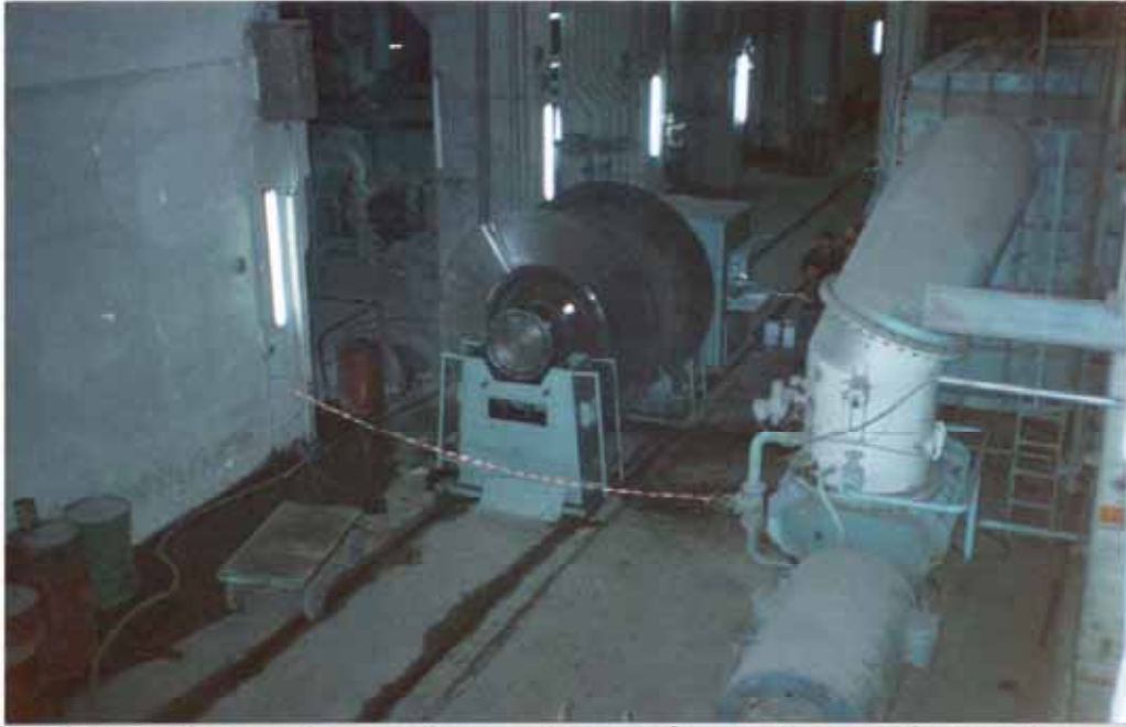
Unit set up in a Power Station on existing track.
